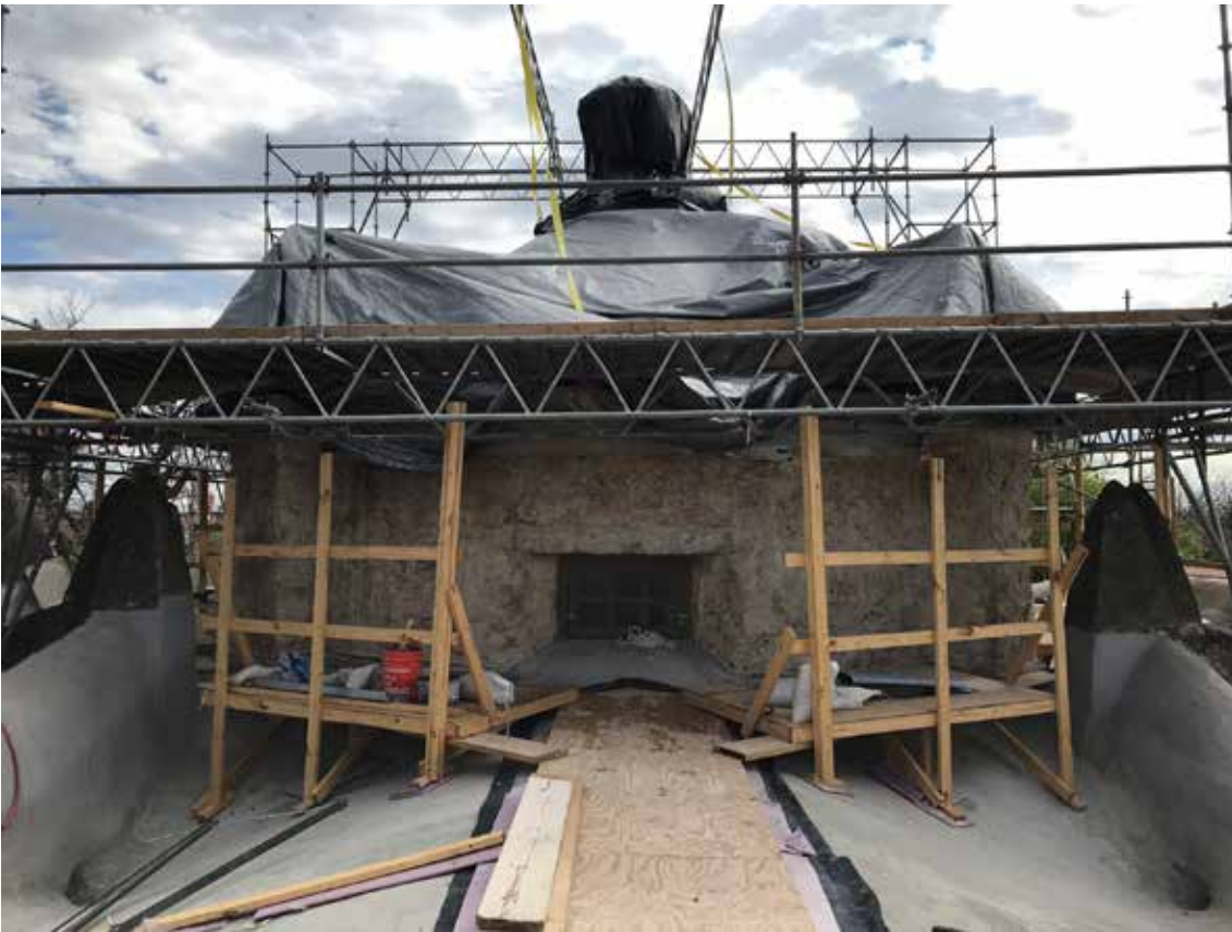
View of west elevation, showing exposed masonry at drum (03.04.2020)
