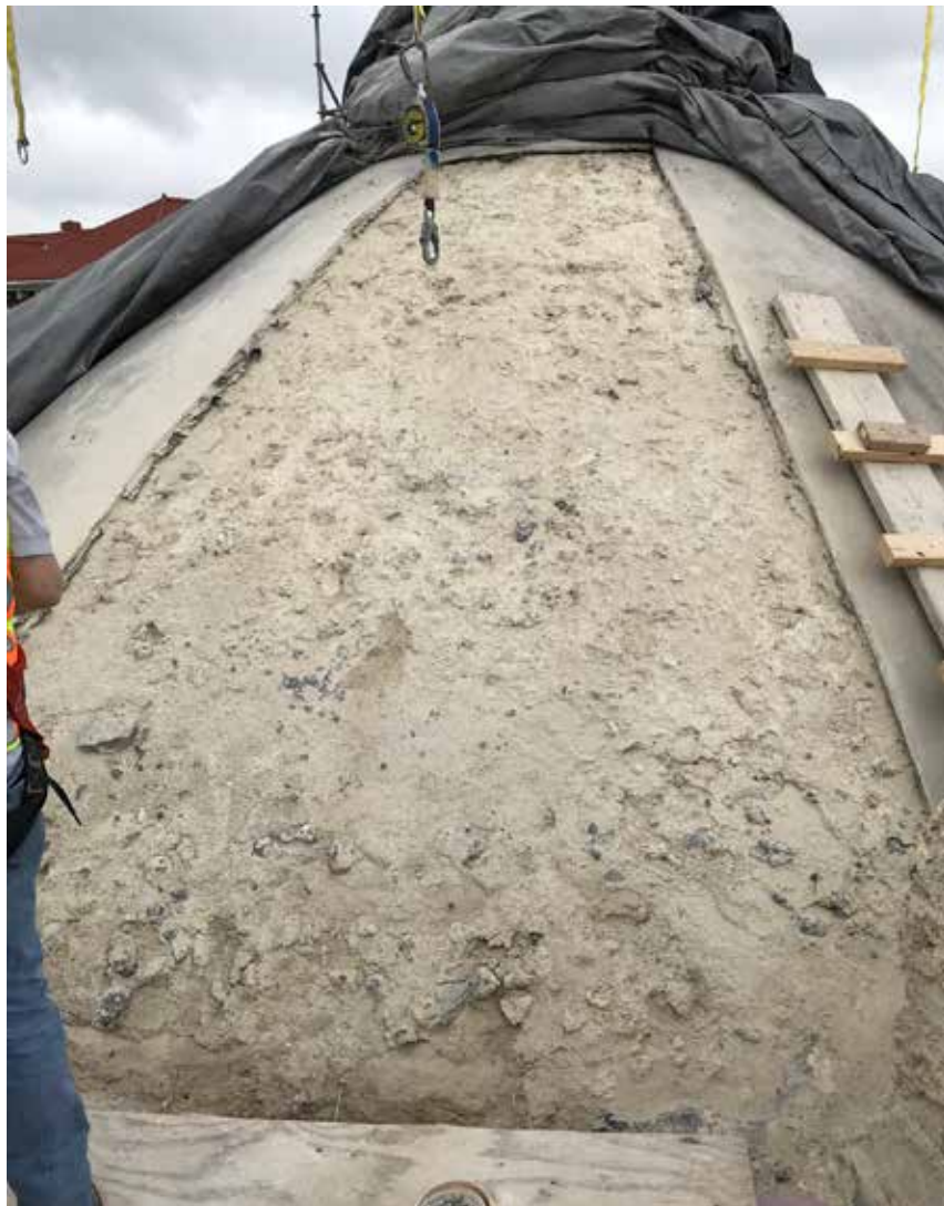
Section of the Dome at the west elevation, after removal of modern roofing materials. This section will receive grout injection and stitching, with stainless steel lath, along the lower 5 feet to help strengthen the stone construction. (03.17.2020)
