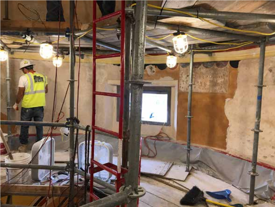
Removal of loose modern plaster at the drum interior (03.16.2020)
