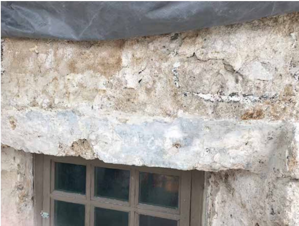
West window at drum, showing area of intact historic Colonial plaster with 19th-century carved graffiti (03.04.2020)
