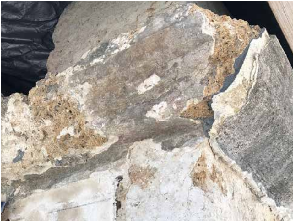
Detail of intact section of historic Colonial plaster at the cornice. This will be used to help us rebuild the historic cornice profile around the perimeter of the dome. (03.11.2020)
