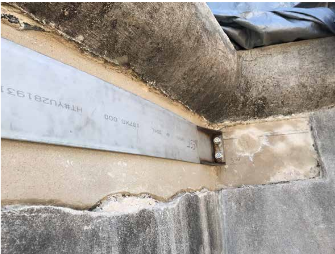
Detail of steel tension band during test fit. Underneath band is a lime plaster "isolation layer" to protect historic mortar and masonry (02.25.2020)
