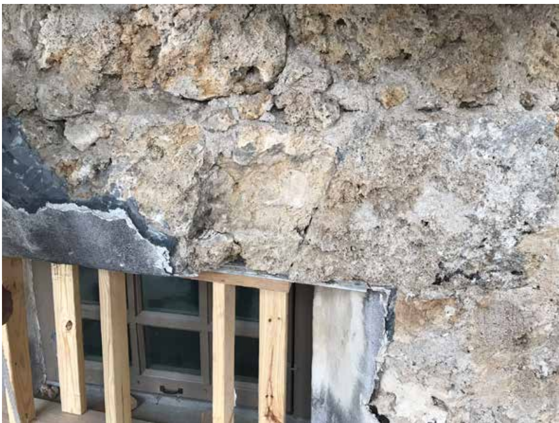
Detail of water damaged mortar and masonry above north window. Hard, dark grey cement (visible at left) from the early 1900s caused moisture to be trapped inside the wall and cause damage. This area has been grouted with mortar and "stitched" with stainless steel rods to strengthen it (03.03.2020)
